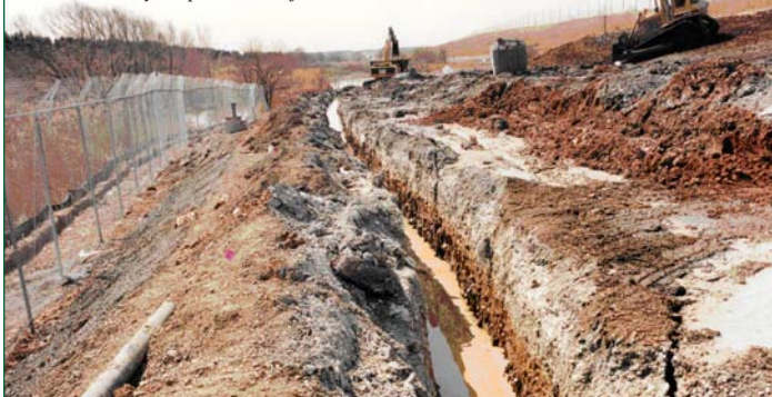
Fresh Kills Landfill Slurry Wall and Site Work, New York City Department of Sanitation.
