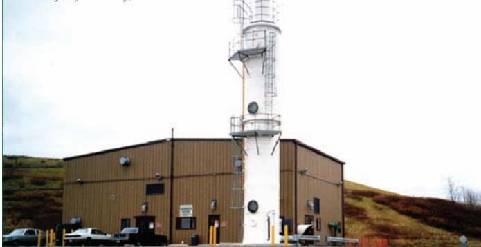
Ground Water Treatment Facility and On-Site Laboratory, Town of Oyster Bay, NY.
